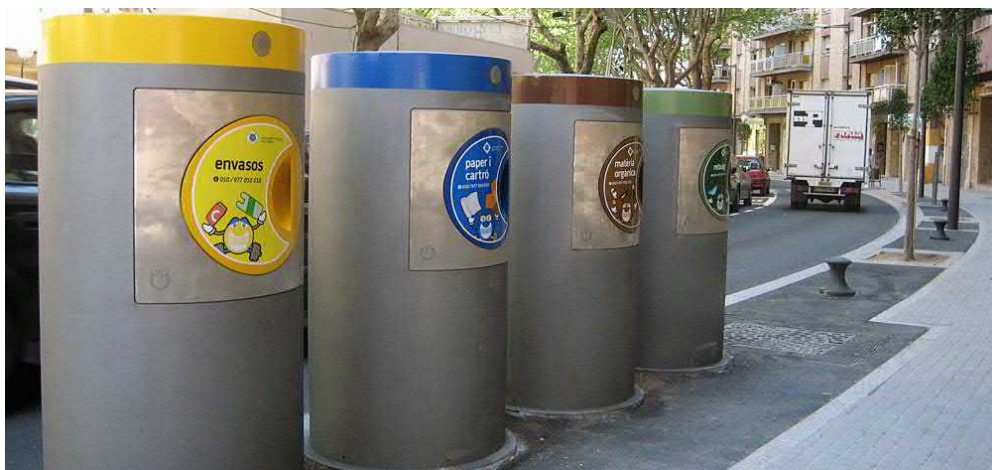
Figure 21: Outdoor waste inlets as part of a precinct vacuum waste collection system
